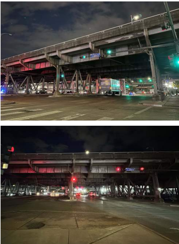
Above: Views of Claiborne underpass at Poydras Street
