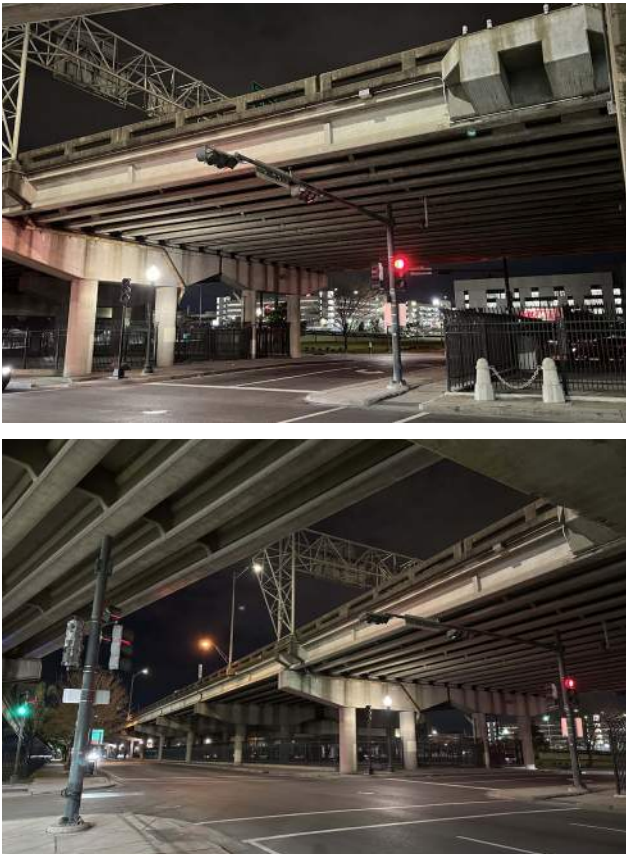
Above: Views of Claiborne underpass at Cleveland Avenue
