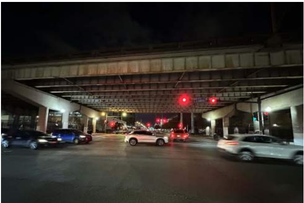
Above: Views of Claiborne underpass at Tulane Avenue
