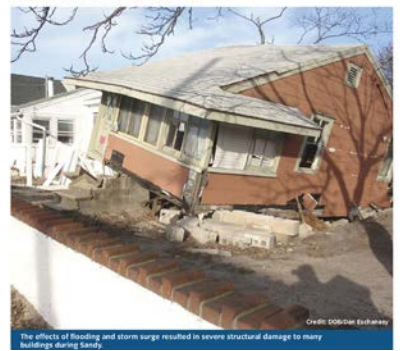
The effects of flooding and storm surge resulted in severe structural damage to many buildings during Sandy. Credit: DOB/DCP/DOB
