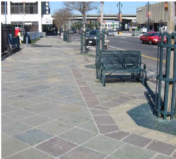
Slate pavers at the Medical Center are in good condition
